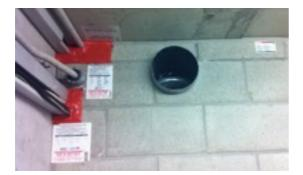
Current day passive fire stopping -installed tested system and properly installed. 当前合理 的防火建设
