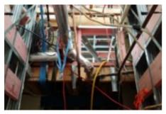
Imagine the impossibility of putting a fire wall through this. 给排水管道, 电缆和暖通管道 系统建设杂乱, 导致防火墙无法铺设
